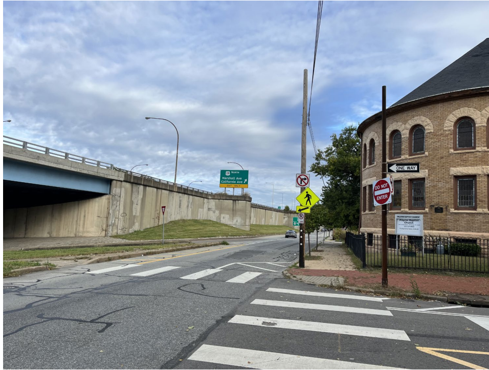
Figure 9. Chateau Street at Juniata Street in Manchester with Route 65 to the west, site of the demolished Manchester School. The Pilgrim (Beth-Eden) Baptist Church as shown on the 1923 map above still stands. (photo: Robert Armstrong, September 27, 2023)
