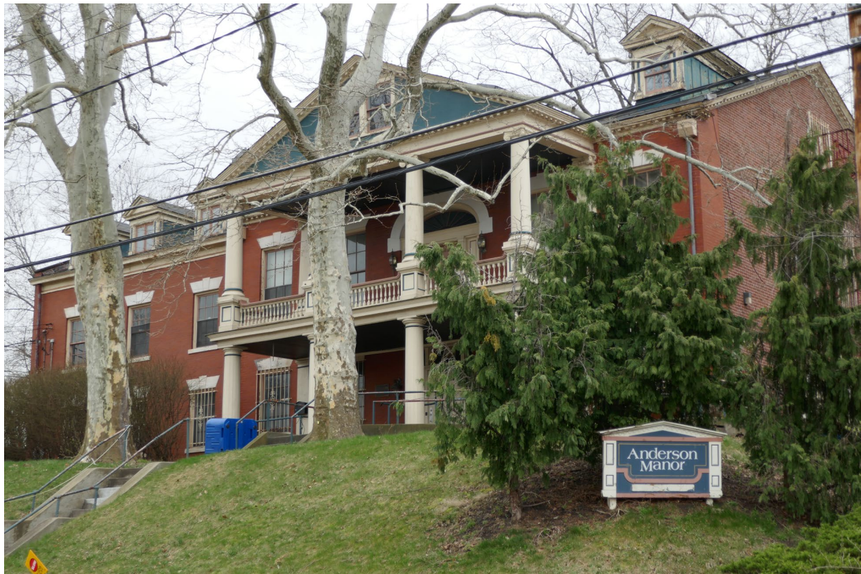
Figure 2. 1423 Liverpool Street, Colonel James Anderson House. Circa 1830 with additions in 1905. (photo: Robert Armstrong, March 27, 2023)
