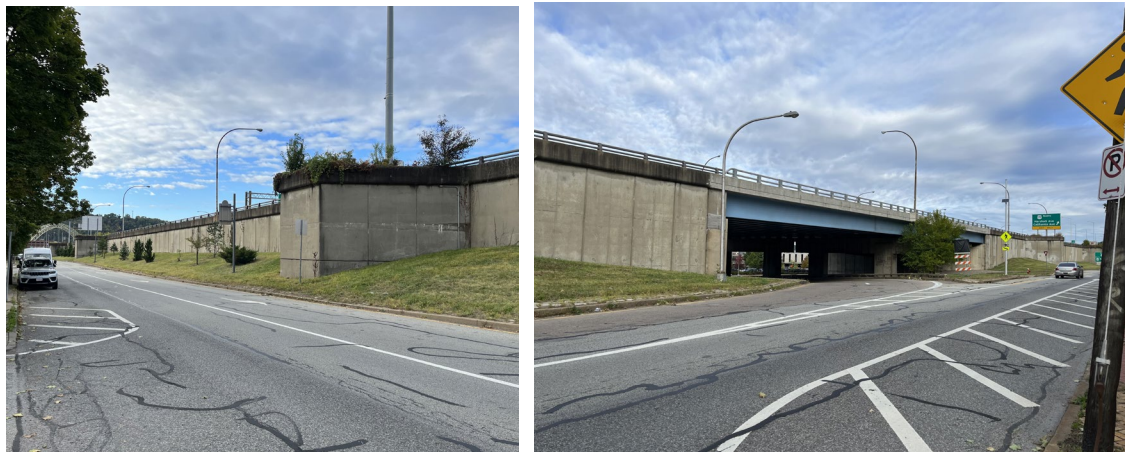
Figure 10. The wall of Route 65 along Chateau Street looking south to the West End Bridge and the only underpass out of Manchester at Juniata Street. During the planning of the highway the District Engineer of State Highway Department stated the Ohio River Boulevard “will either be elevated or depressed so that present street patterns will remain intact.” 18 Instead, present major east-west streets terminated at the wall and the neighborhood was divided on a north-south axis. (photo: Robert Armstrong, September 27, 2023)
