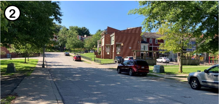
There are no ADA curb ramps or crosswalks at main entrance along Wilner Drive.
