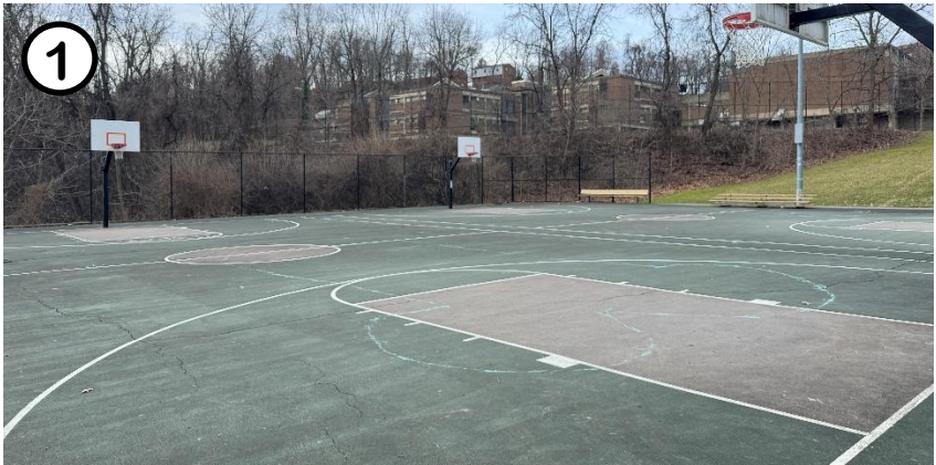
Existing courts can be improved by resurfacing.
