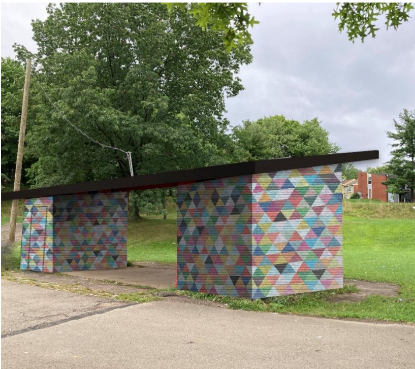
Mural on Existing Shelter
