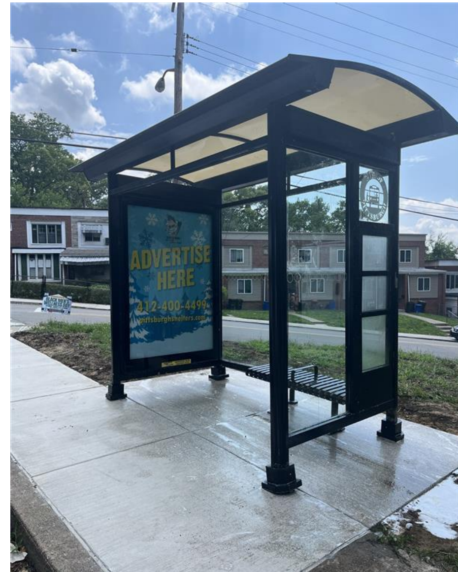
Hamilton Ave & Oakwood St
