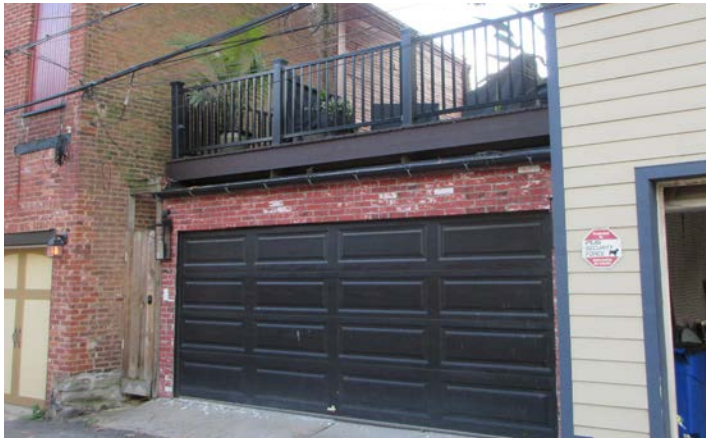
Appropriate roof deck on noncontributing accessory structure
