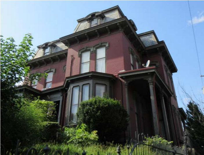
Some detached residences have associated landscape features, including retaining walls and fences
