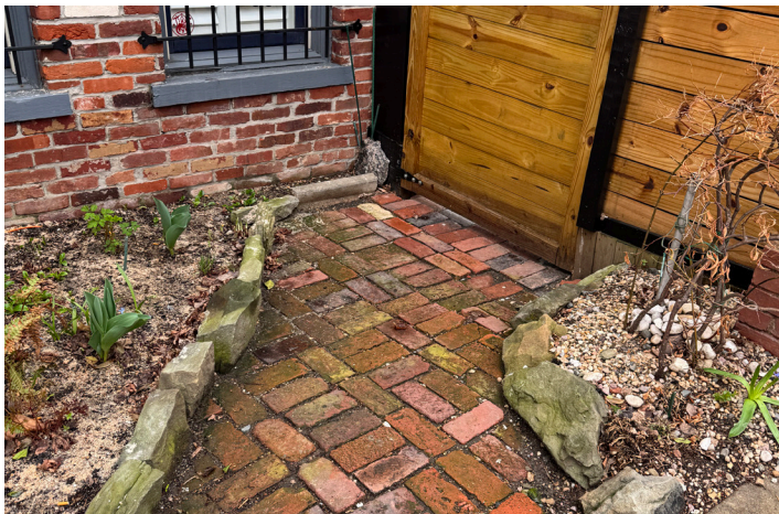
Brick is an appropriate material for walkways.
