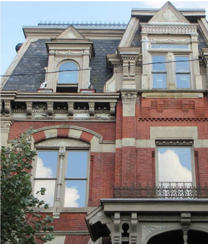
Retain original windows when possible.
