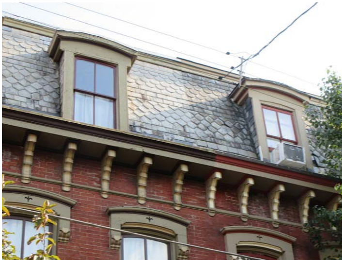
This mansard roof with multiple slate patterns is both durable and decorative
