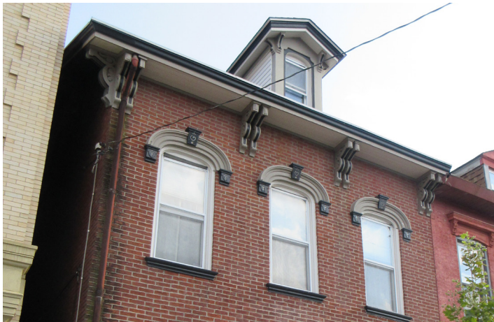
Historic built in gutters and metal downspouts.
