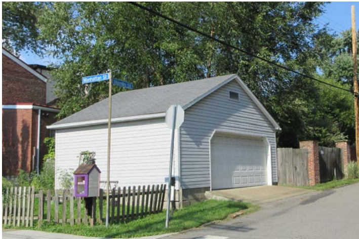
Noncontributing accessory structures are those built outside of the period of significance for the historic district, and do not contribute to the historic fabric of the district.
