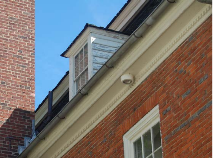
Modern facade lighting is concealed under the eave and the fixture color blends in; this is an appropriate installation.
