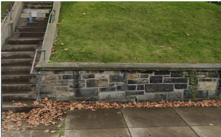
Preserved historic masonry retaining wall..
