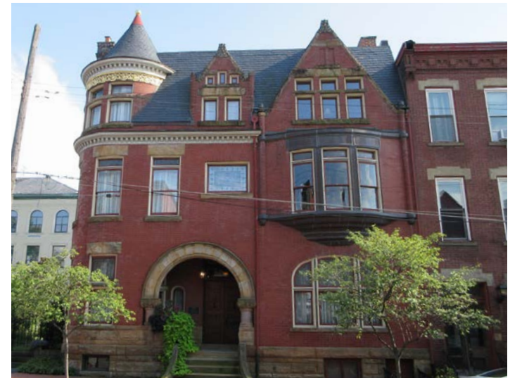
Romanesque Revival facade with wall dormers, corner turret, and multiple rounded elements
