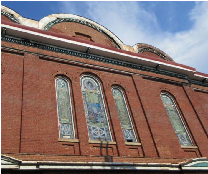
Retain original character windows when possible.
