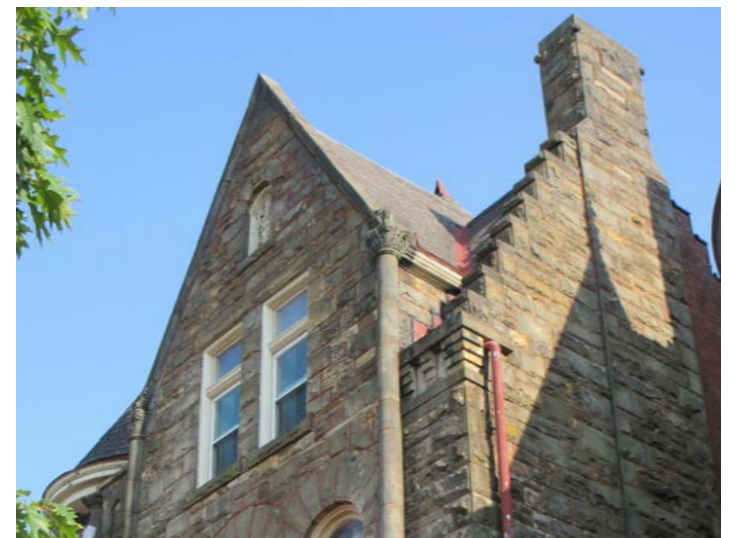
Quarry-faced sandstone construction characteristic of the Romanesque Revival style
