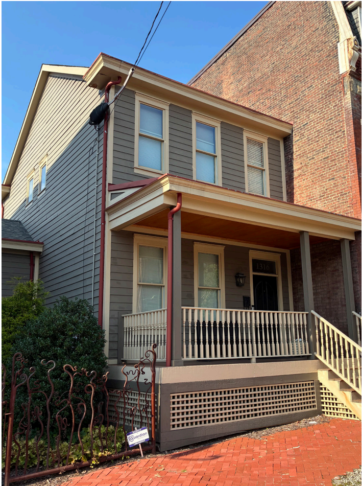
Preserved original wood siding and trim.
