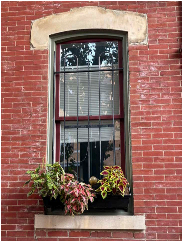
Example of appropriate window grill configuration.
