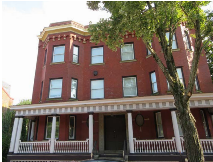
Three-story Colonial Revival double house with symmetrical bay windows and continuous front porch
