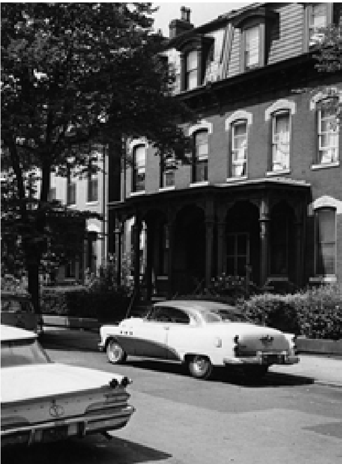
Photo: Historic facades on 1300 block of Liverpool Street circa 1966 (Pittsburgh History & Landmarks Foundation Website)
