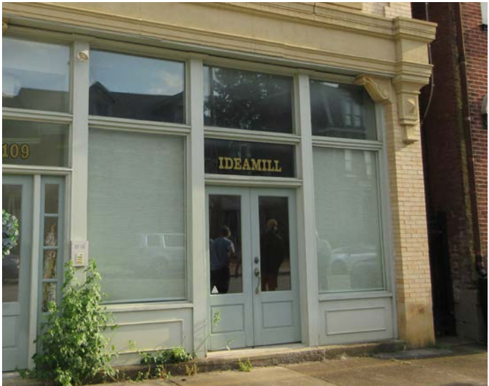
Historic storefront that utilizes historic painted window signage for business identification.
