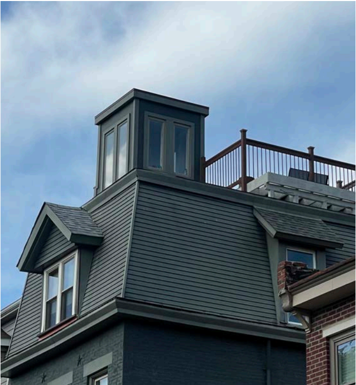
Example of inappropriate addition in massing, scale and location.
