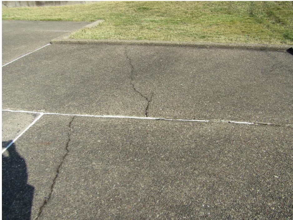
Figure 3.b-3: Typical cracks.
