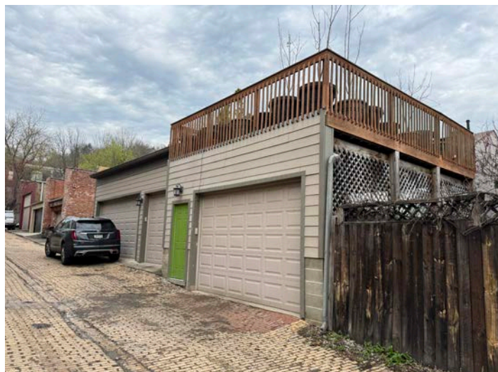
Appropriate roof deck on noncontributing accessory structure
