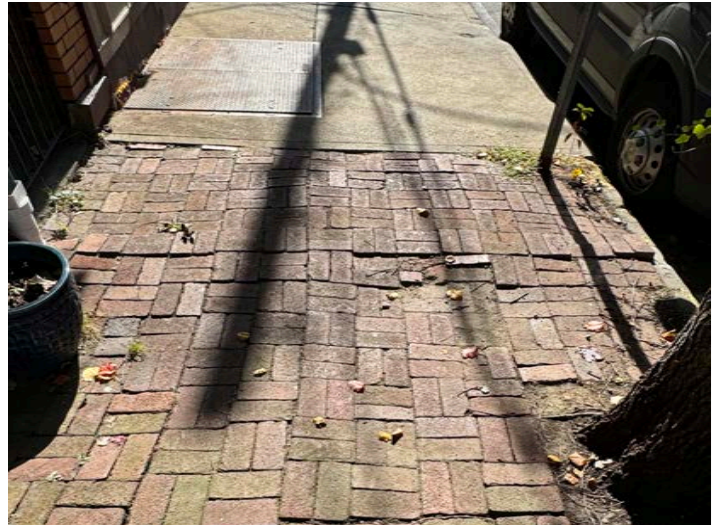
Existing brick sidewalks should be maintained.
