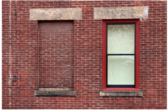
Example of appropriate window infill on a non-primary facade.
