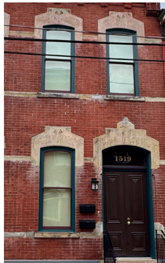
Windows with flush lintels
