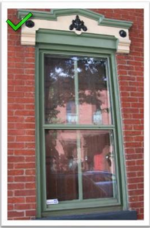
An exterior storm window protects the original wood sashes from the elements. This storm window is not a perfect fit for the opening but is well disguised with matching paint colors.
