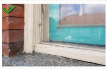
This exterior storm window fits snugly within the window frame and is minimally visible.
