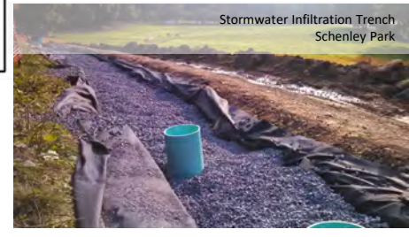
Subsurface Storage Stone
