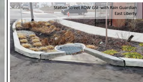
Debris Capture Inlets
