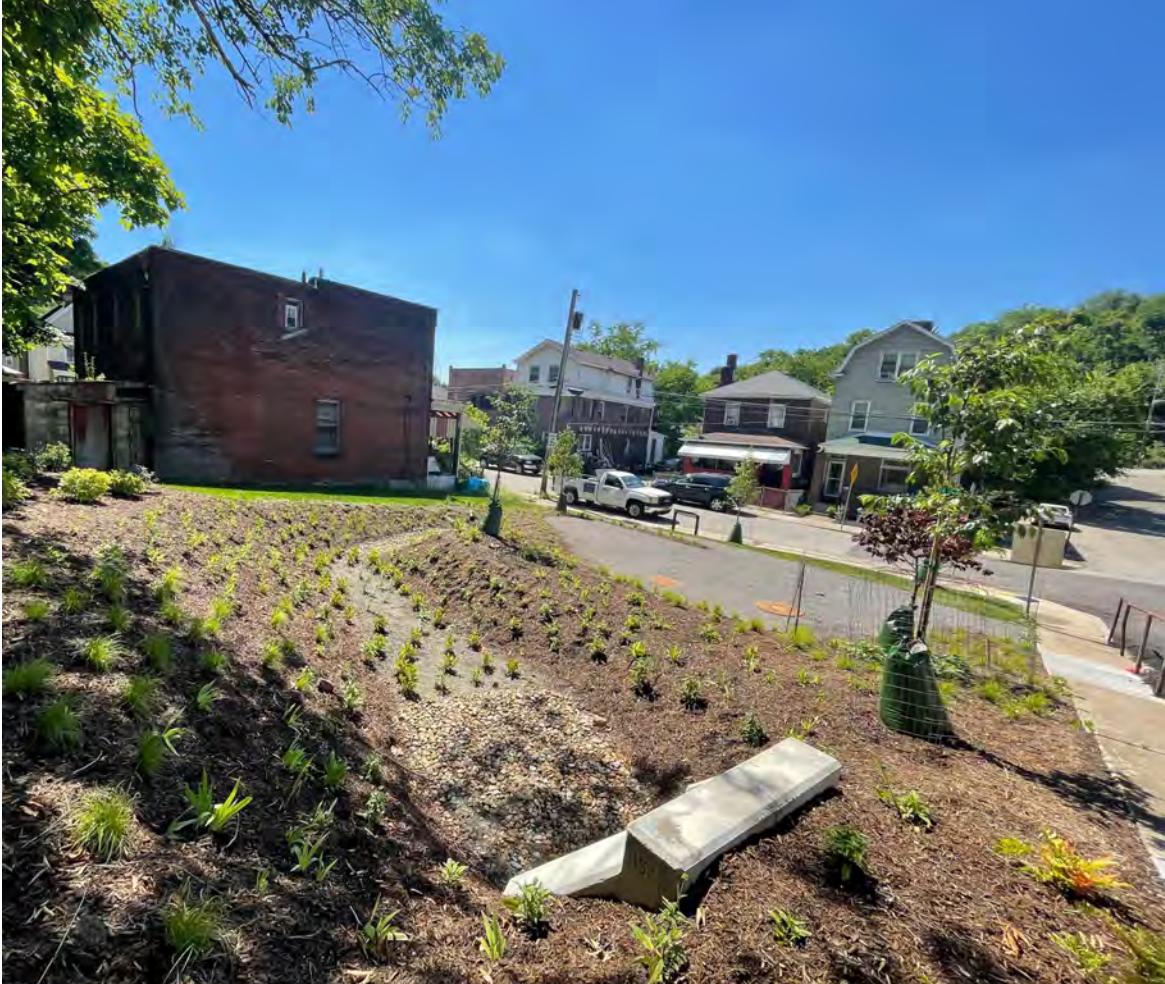
Dornbush Green Infrastructure Project (after construction), Upstream Pittsburgh
