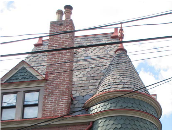
Historic slate roofing
