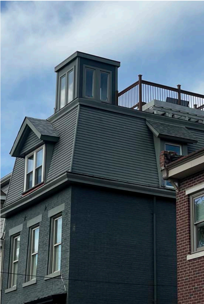
Example of additions inappropriate in massing, scale and location.
