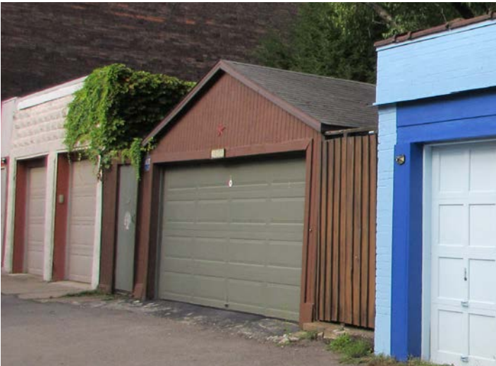
Appropriate new architectural element.
