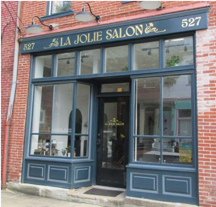
Historic storefront with appropriate signage.
