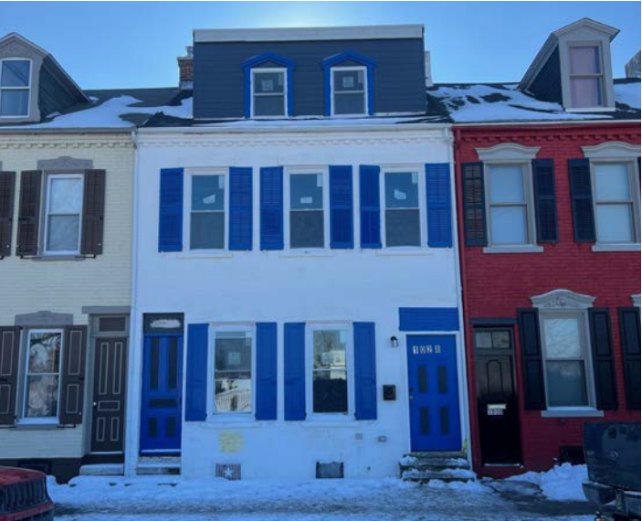
Example of an inappropriate dormer addition, which removed an original dormer and created non-historic proportions.
