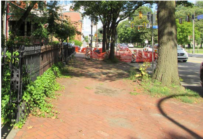
Existing brick sidewalks should be maintained.
