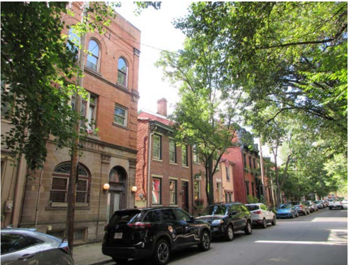
A variety of façades forms the streetscape of the historic district.
