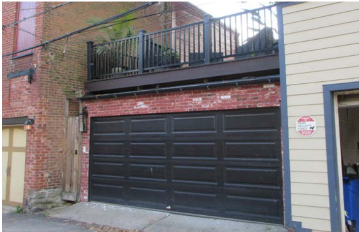
Appropriate roof deck on noncontributing accessory structure
