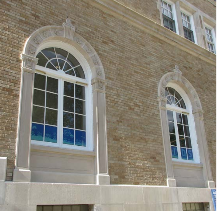
Retain original windows when possible.
