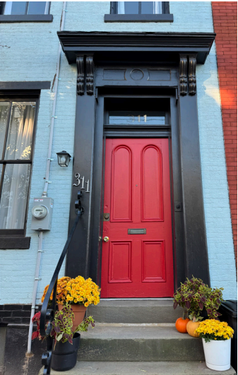
Inappropriate example of a meter located on a primary facade.
