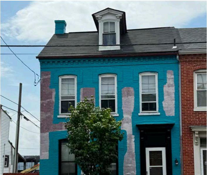
Example of inappropriate use of paint on masonry substrates.
