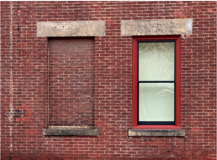
Example of appropriate window infill on a non-primary facade.
