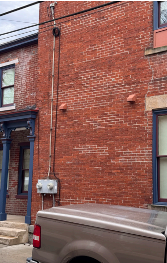
Appropriate example of a meter and vents placed on secondary facade.
