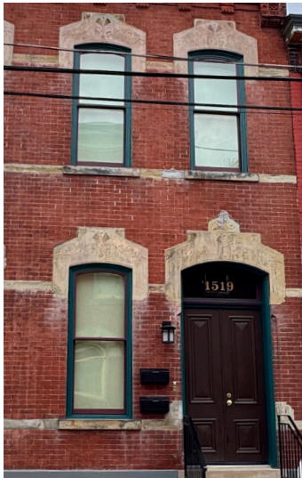
Windows with flush lintels
