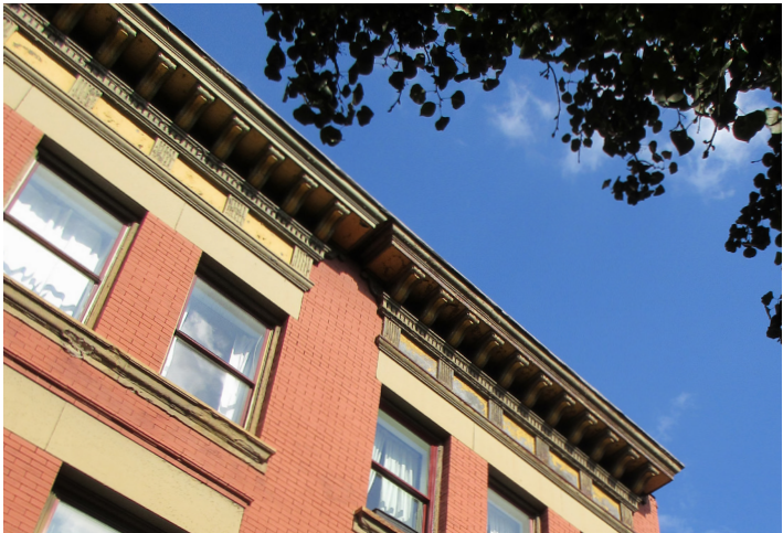
historic cornice at a flat roof.
