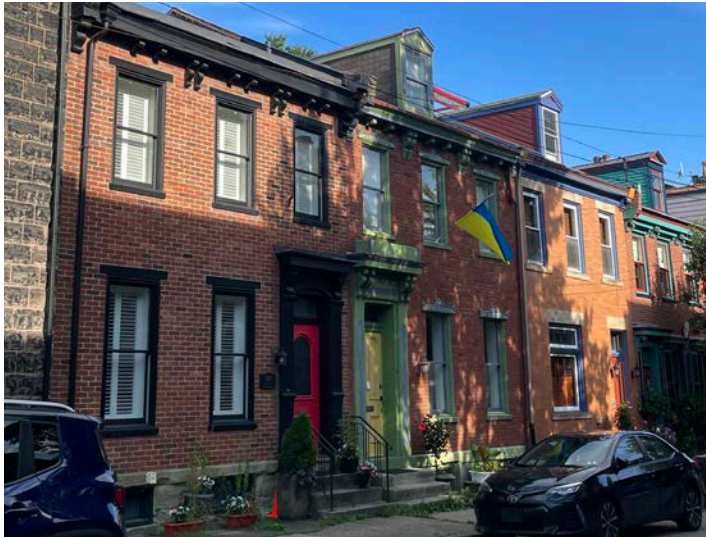
Example of Historic District façades composition.
