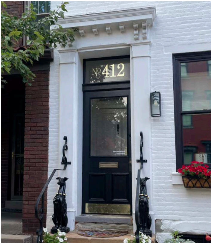
Appropriate new metal railing element.
