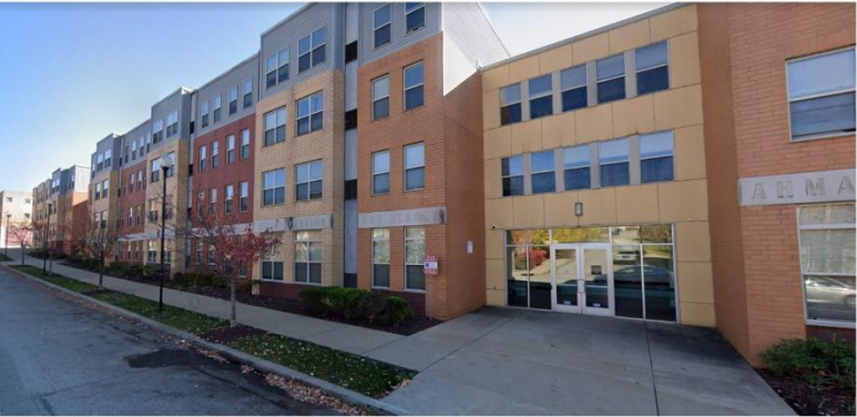
CONTEMPORARY WITH CENTRALIZED LOBBY AND NARROW SETBACK
