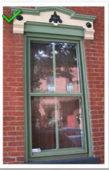
An exterior storm window protects the original wood sashes from the elements. This storm window is not a perfect fit for the opening but is well disguised with matching paint colors.
