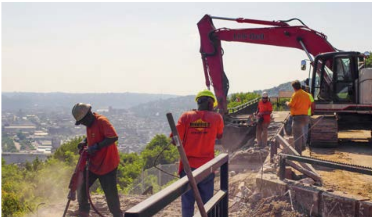
Repair of an elevated sidewalk platform between Maple Terrace and Shiloh Street
