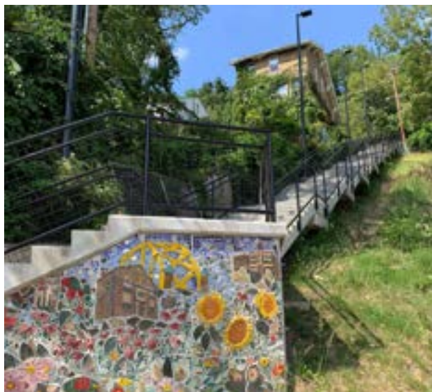
The newly reconstructed Vista Street Steps on the North Side.
