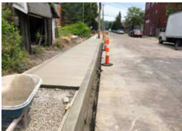
Recent critical sidewalk gap construction
