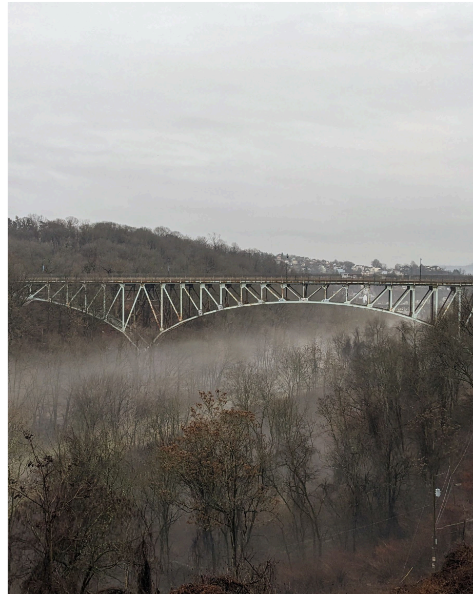
Charles Anderson Bridge
