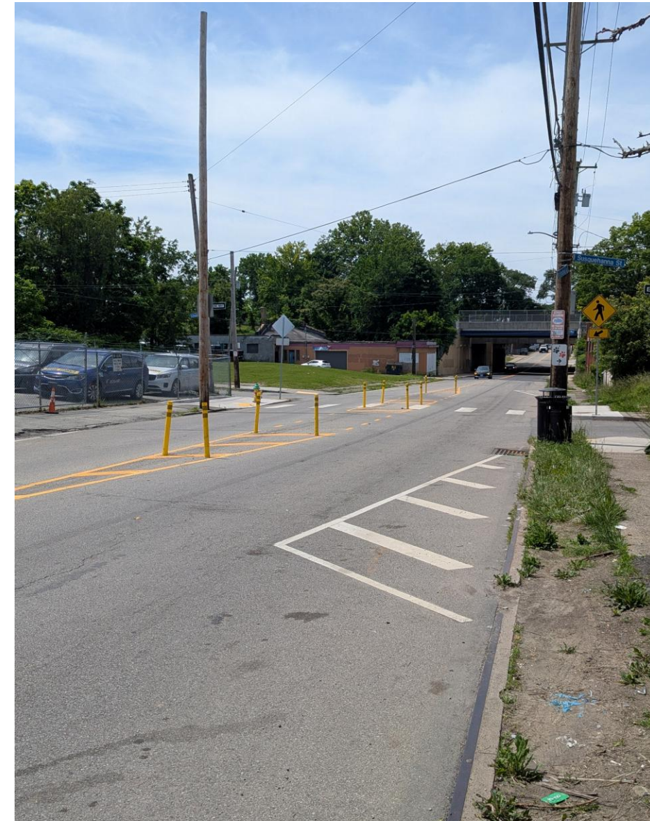
Braddock Avenue- Susquehanna St. Crossing Improvement
