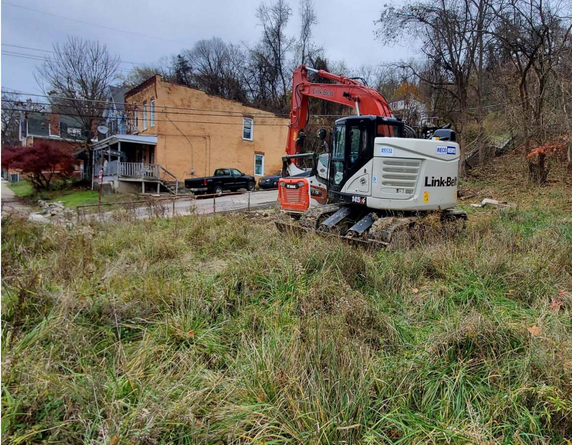
Dornbush Green Infrastructure Project (before construction), Upstream Pittsburgh
