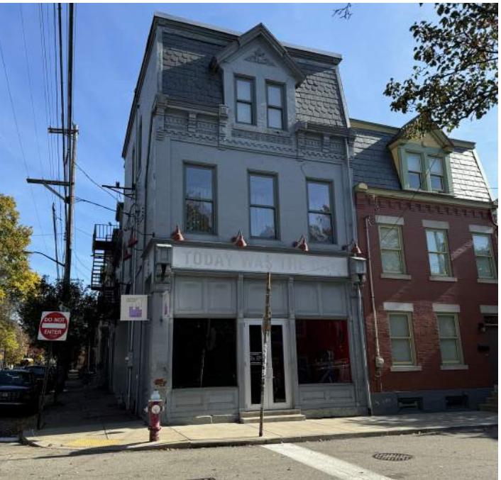
Historic storefront with wood panels, detailing, and signboard.
