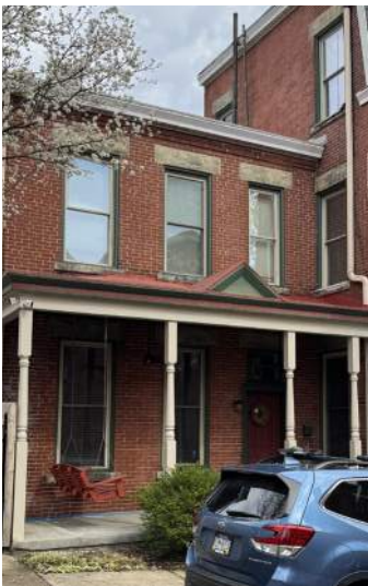
Metal roof at porch.
