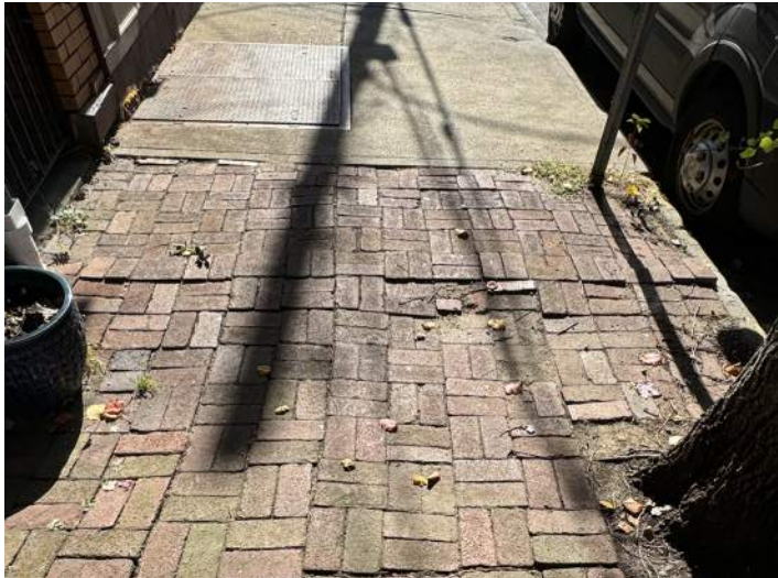
Existing brick sidewalks should be maintained.
