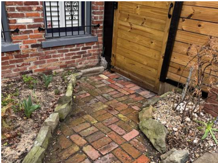
Brick is an appropriate material for walkways.
