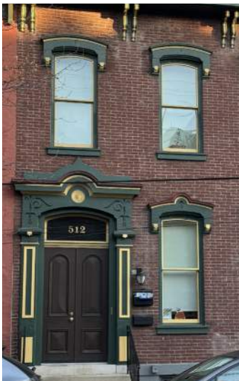
Windows with projecting hoods
