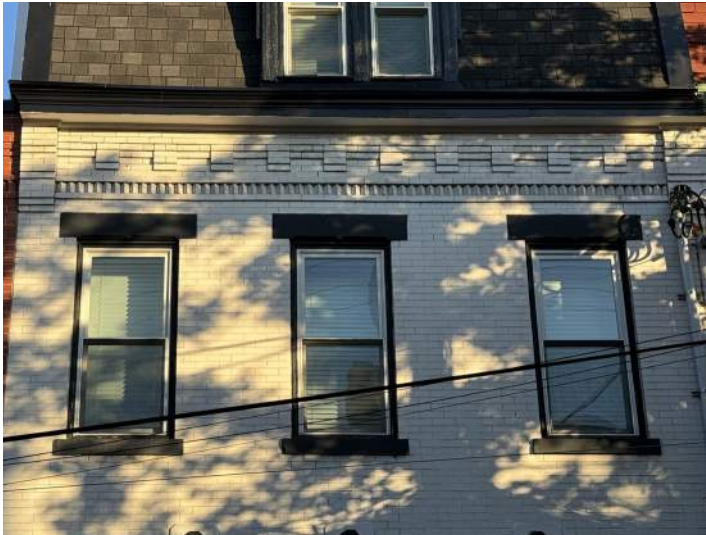
Running bond is typical on this wall, and features decorative brick pattern at the cornice.
