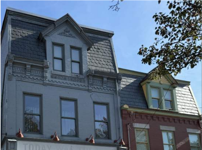
Existing slate mansard roofs retain historic character and should be retained.
