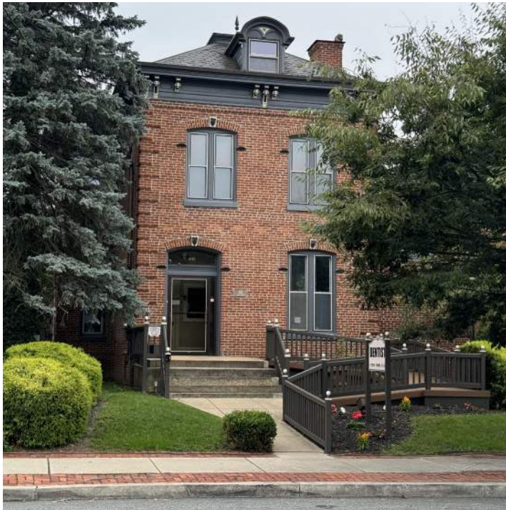
Example of an appropriate accessible entry modification.
