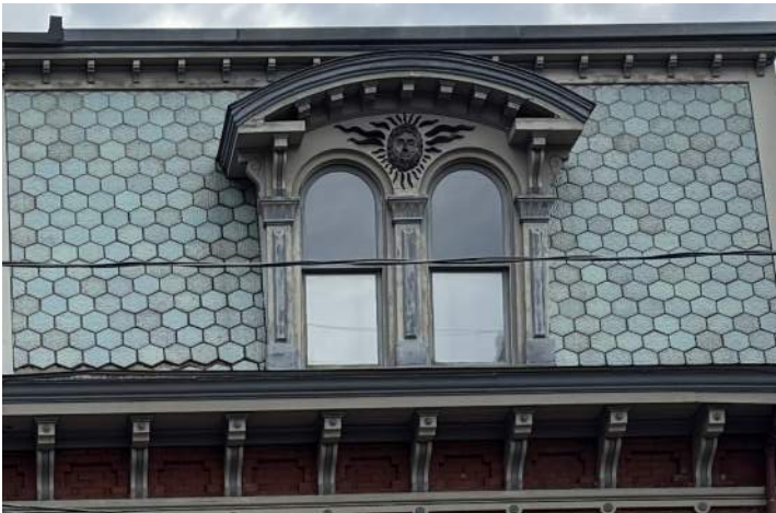
Retain original windows when possible.
