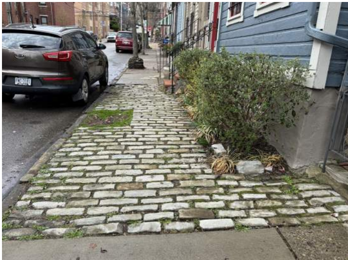
Existing cobblestone sidewalk.
