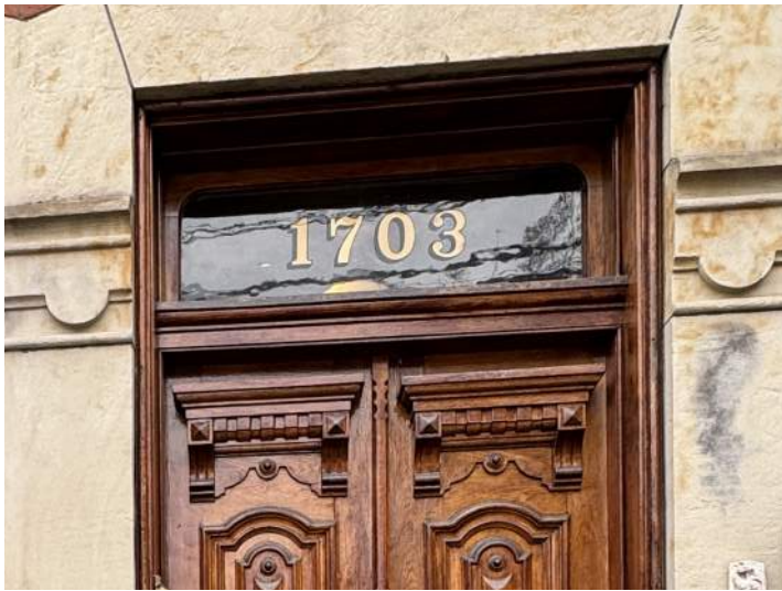
Appropriate address label in doorway transom.
