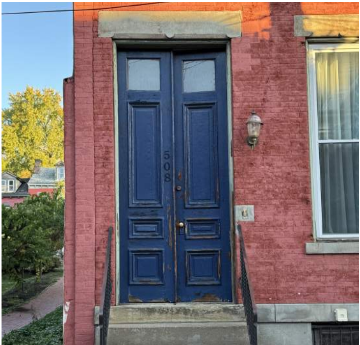
Historic wood doors should be maintained.
