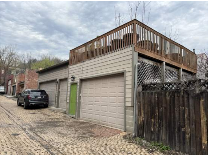
A roof deck may be appropriate on a noncontributing accessory structure, such as a garage.
