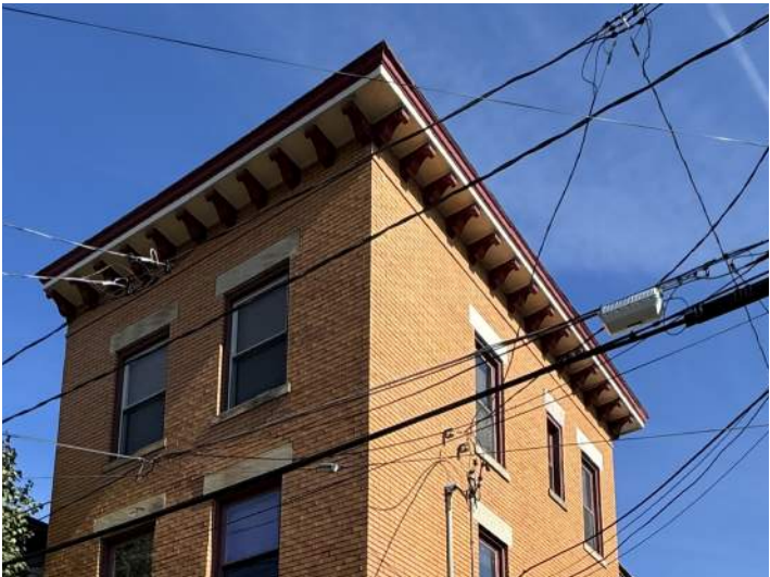
Existing decorative cornice at a flat roof.
