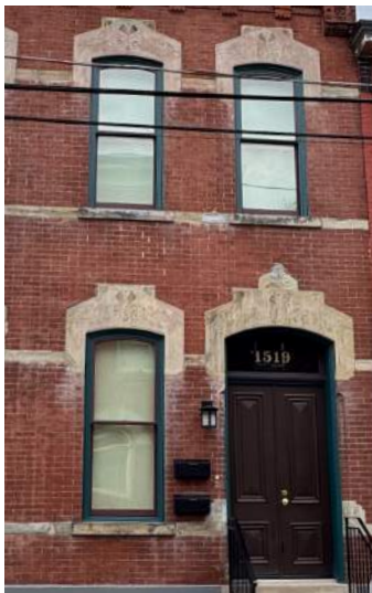
Windows with flush lintels
