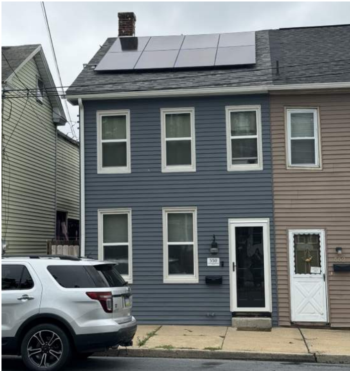
Example of inappropriate solar panel installation on roof slope easily seen from a right-of-way.
