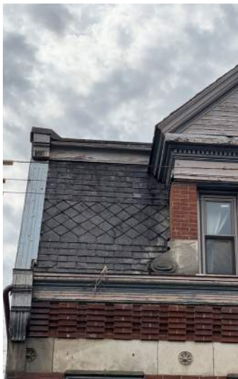
Slate mansard roof, featuring various patterns.
