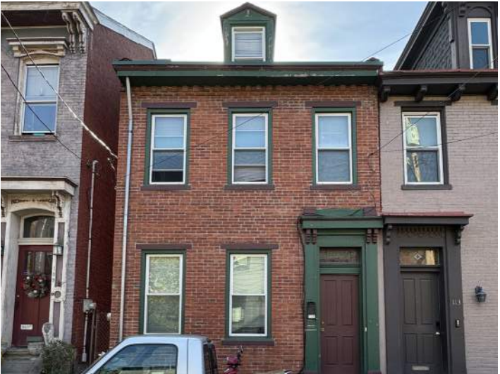
Existing built-in gutters with metal downspouts.
