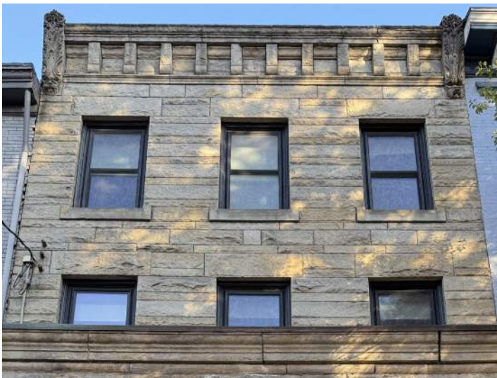
Stone masonry used as the overall facade material of this Romanesque style building.
