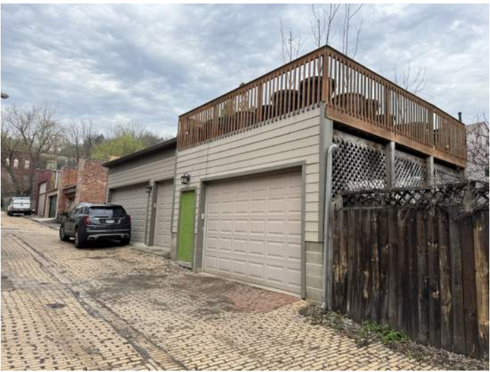
Properties commonly extend to alleys, and may have an accessory structure, such as a garage.
