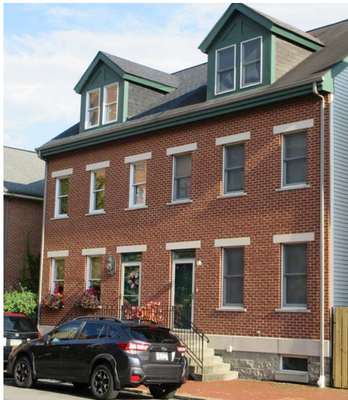
Appropriate new construction materials.
