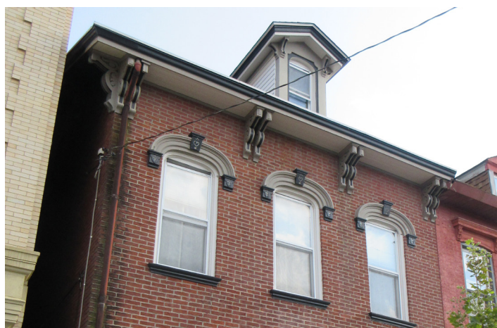
Historic built in gutters and metal downspouts.
