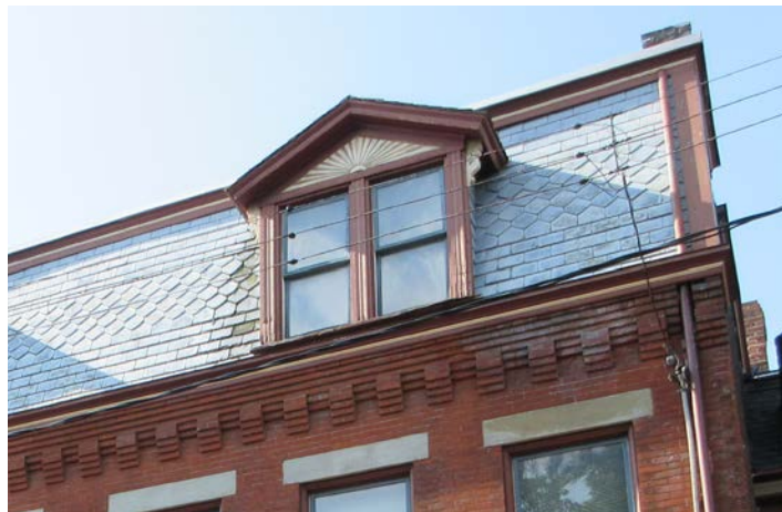
Historic slate roofing
