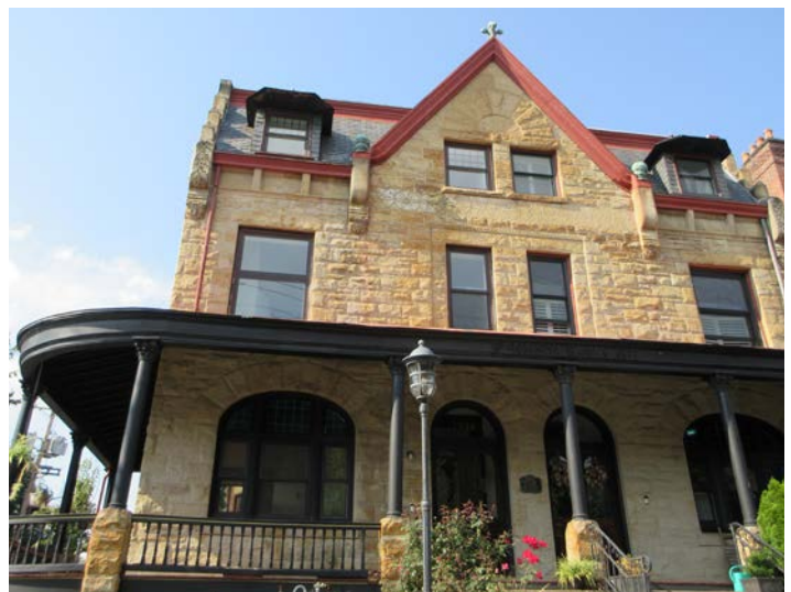
The corner location of this house allows for a wraparound porch
