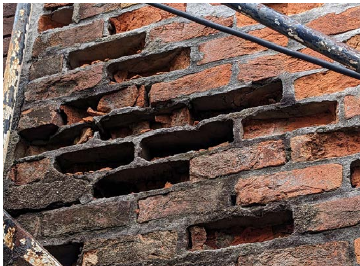
Example of deterioration to masonry caused by inappropriate strength mortar repair.
