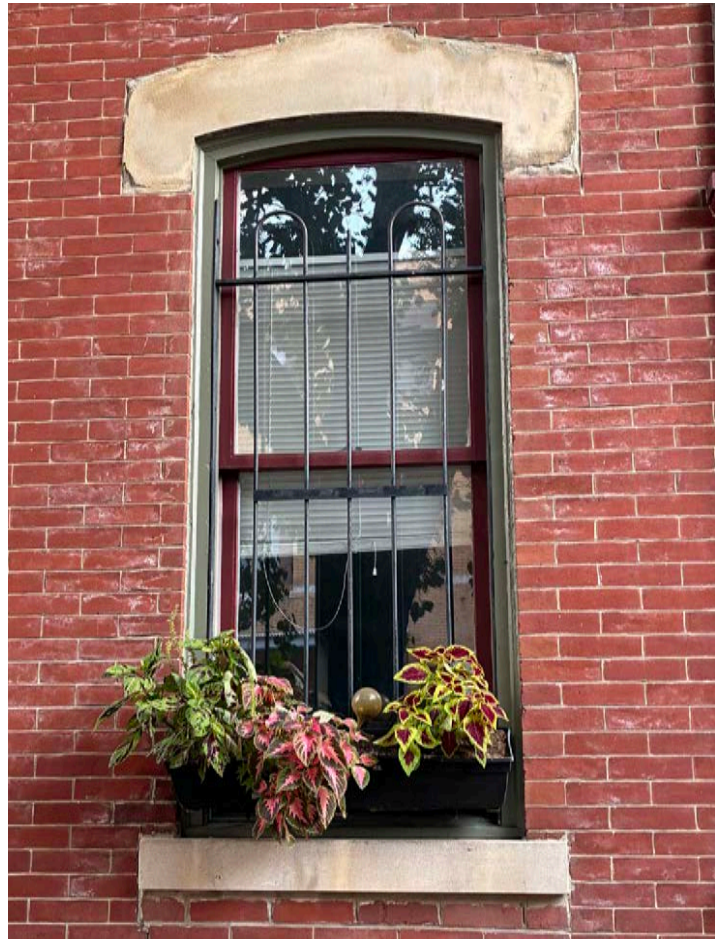
Example of appropriate window grill configuration.
