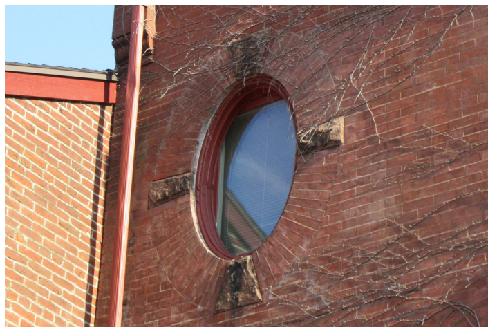
Example of replacement window that is not appropriate (square window in a round opening).
