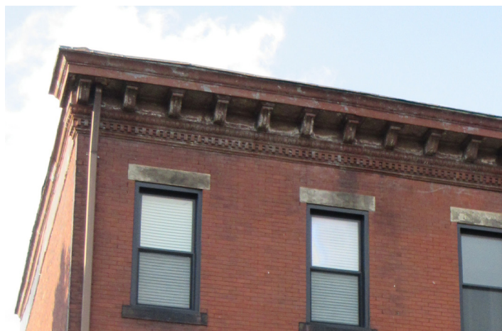
Historic cornice at a flat roof.
