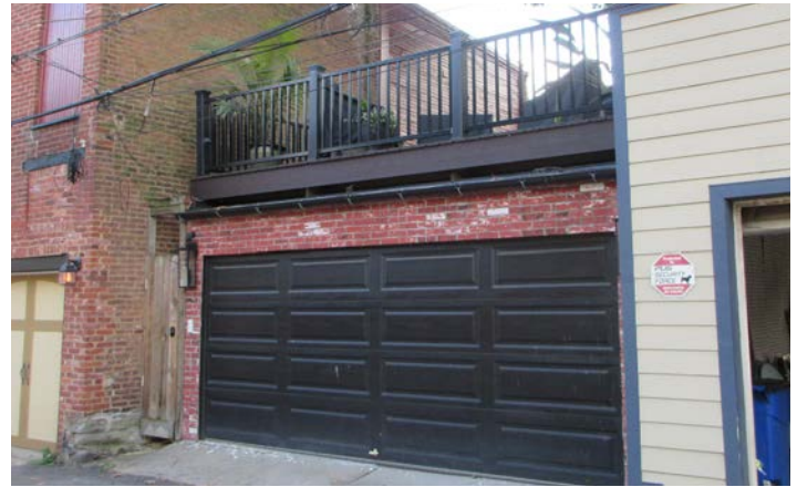
Appropriate roof deck on noncontributing accessory structure
