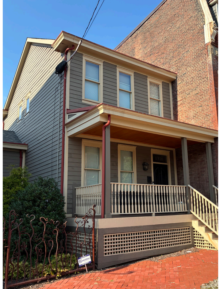
Preserved original wood siding and trim.
