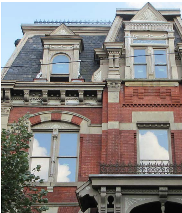
Retain original windows when possible.
