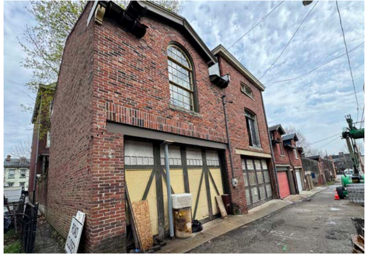
Appropriate accessory structure.
