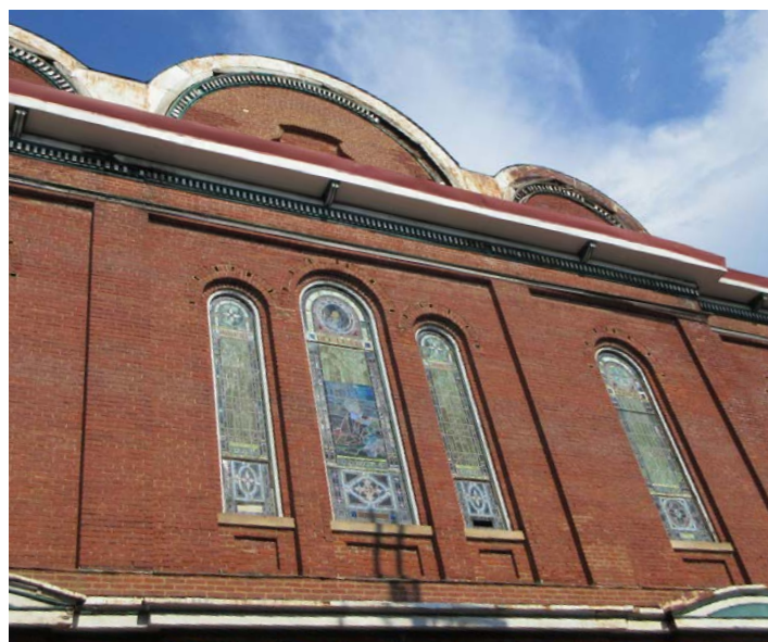
Retain original character windows when possible.
