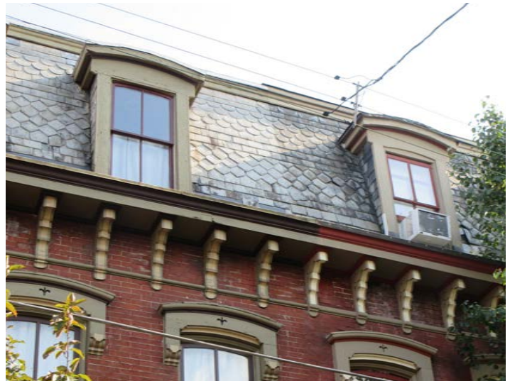
This mansard roof with multiple slate patterns is both durable and decorative
