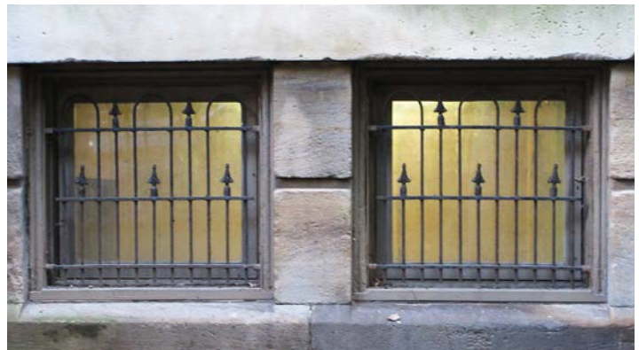
Example of appropriate window grill configuration.
