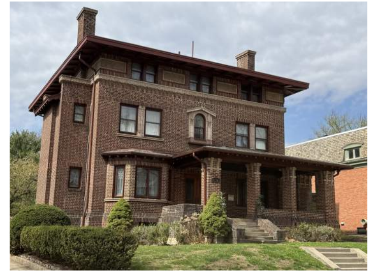
An example of detailed masonry construction.
