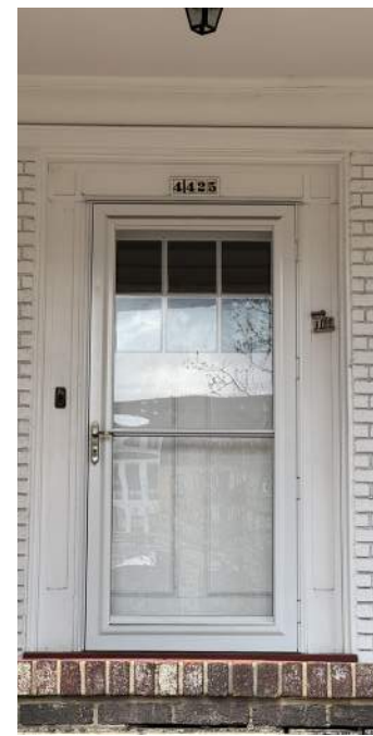
Full view storm doors offer protection for original doors.
