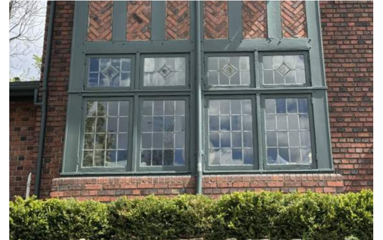
Retain original windows when possible.
