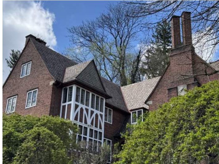
Existing slate roofs retain historic character and should be retained.
