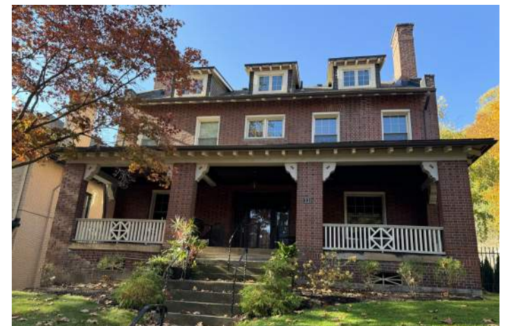
Porches are typically supported by wood or masonry columns.
