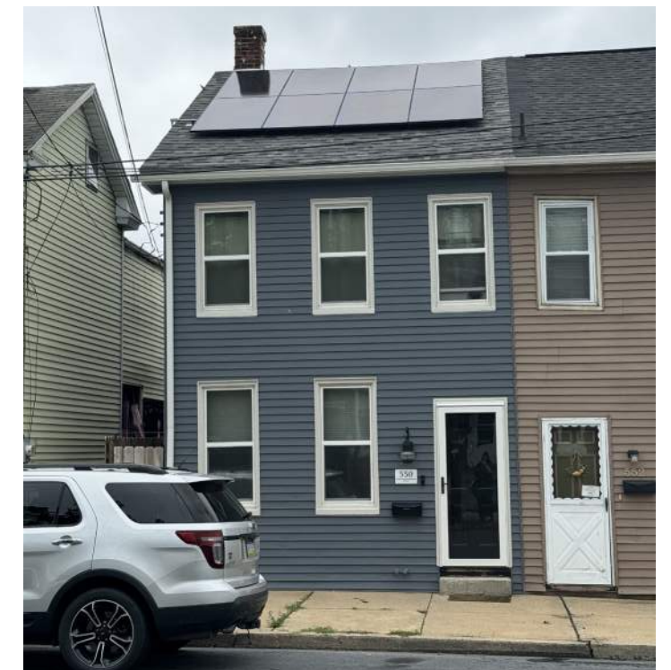
Example of inappropriate solar panel installation on roof slope easily seen from a right-of-way along the primary elevation.
