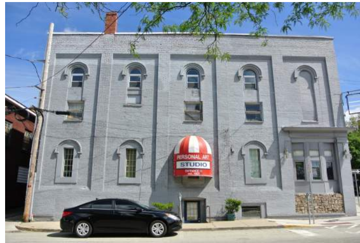
Example of replacement windows that are not appropriate.
