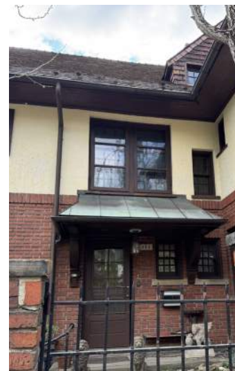
An example of a slate roof and metal entry hood.
