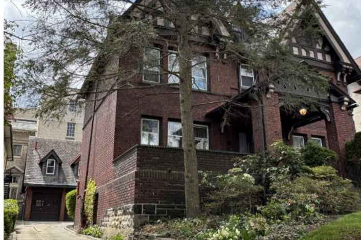
Accessory structures are considered contributing when they carry their own architectural significance. Often, historic accessory structures have similar detailing as the main structure.
