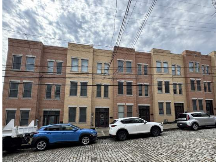
Example of new construction following rhythm and form of the surrounding historic streetscape.
