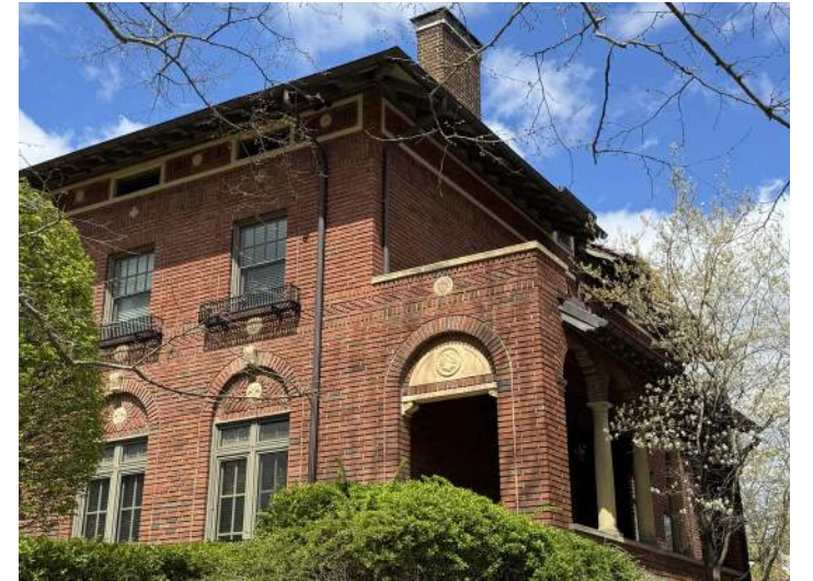
Masonry and wood elements should be maintained to ensure their longevity.
