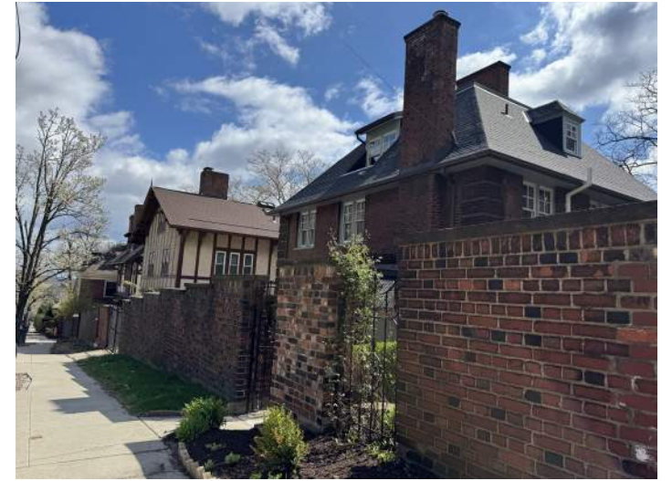
Existing brick fence with iron gates.
