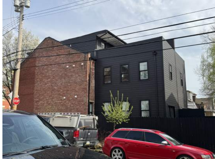
Example of appropriate massing and location of an addition at the rear of a property.
