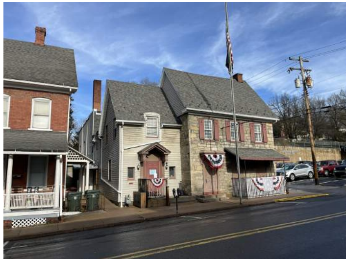
Example of an appropriate addition, which has similar proportions and roof slopes, but is smaller than the original structure.
