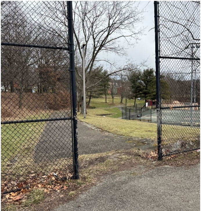
Existing Conditions – Location B
