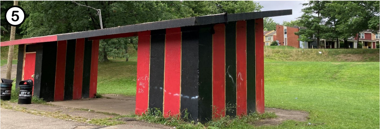
The pavilion houses electrical equipment. The shelter must remain or provisions will be necessary to house or relocate electrical equipment.
