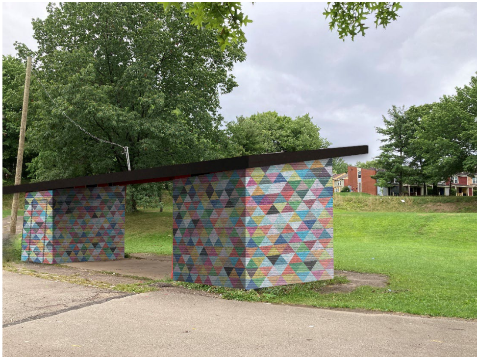
Mural on Existing Shelter
