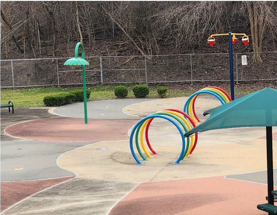
Repairs to Existing Spray Park Features
