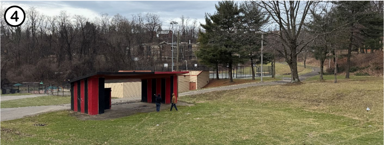
Existing pavilion and open lawn could be improved for community events.
