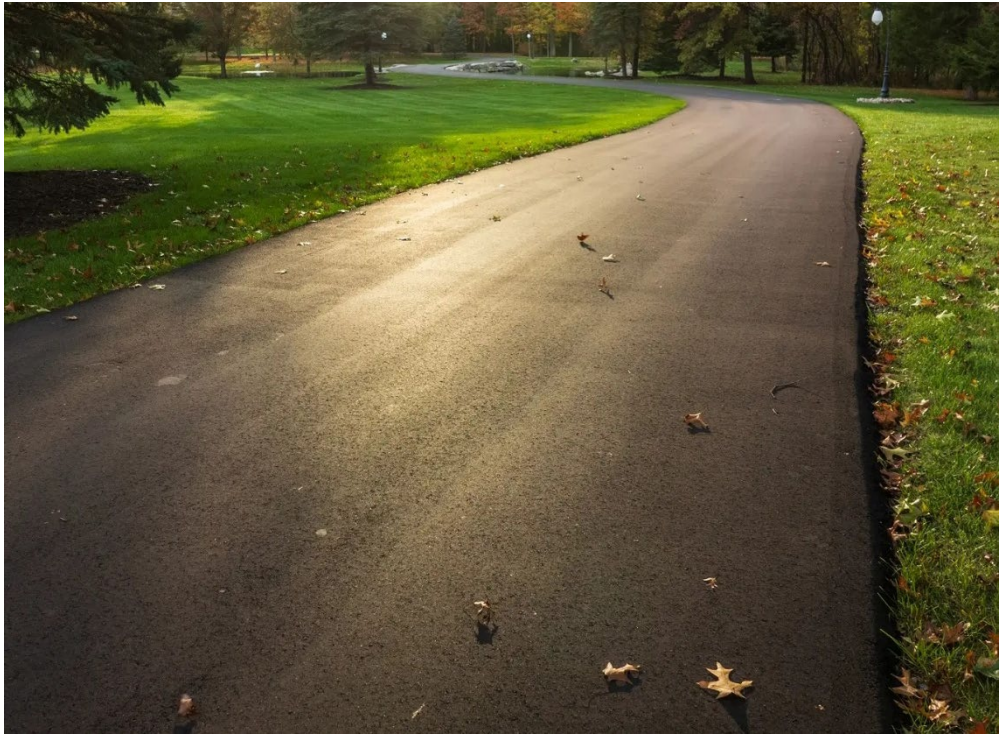
Repave Park Pathways
