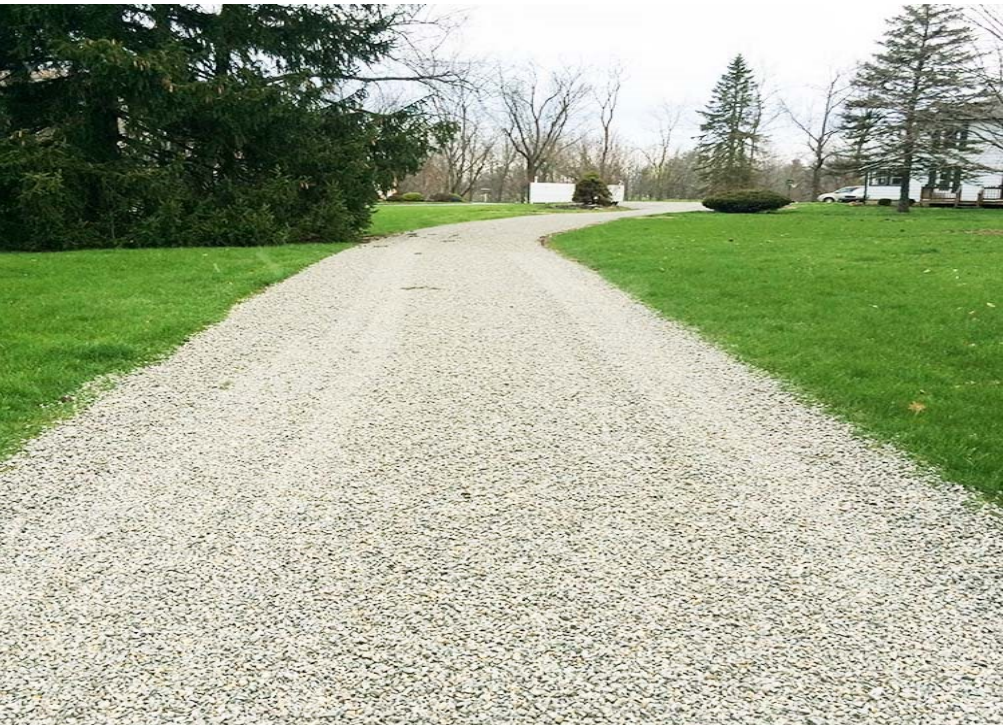
Crushed Stone Walking Path (Around Perimeter)
