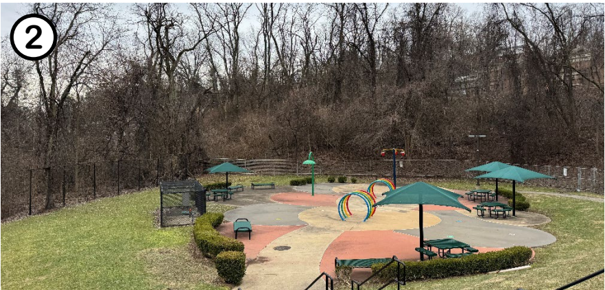
Spray park can be repaired and improved by replacement of site furnishings
