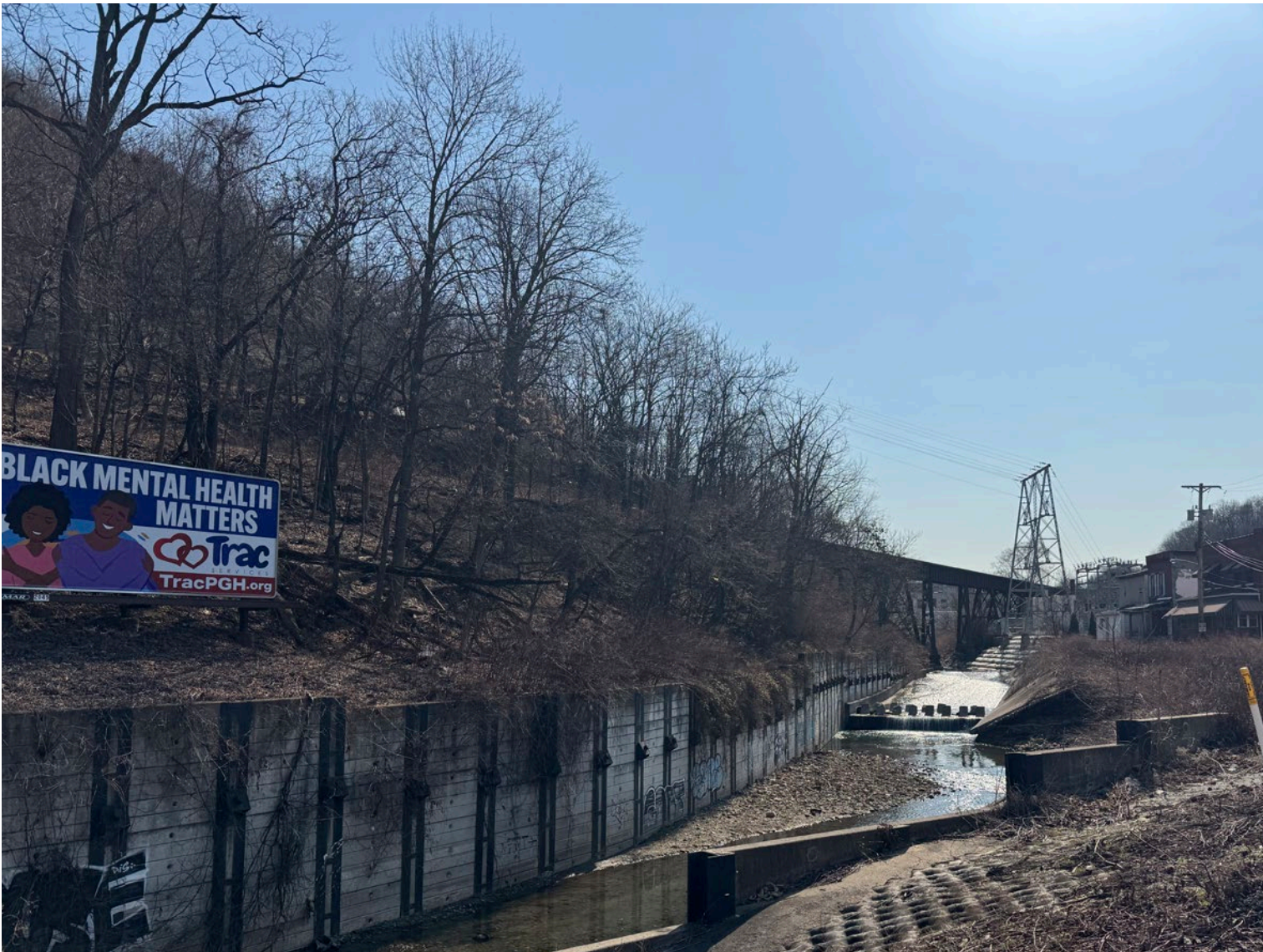
Saw Mill Run and Rail Road Trestle
