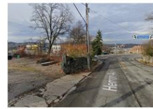
DISCONNECTED STREET EDGE AT HERRON AVE AND BIGELOW BLVD
